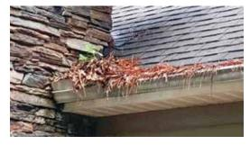
Clogged gutters and downspouts will cause water to overflow. This overflow could cause fascia rot, amongst other costly issues.
